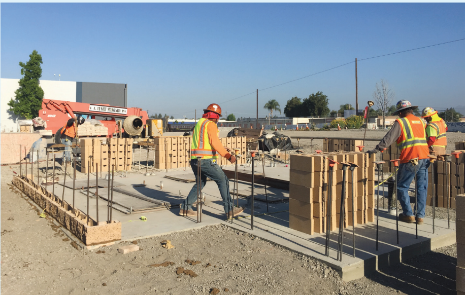
Crews construct the pump station for the Fairway Drive grade separation project that will improve drainage and remove stormwater from the future roadway underpass.
