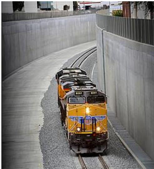
USA: A 2.3 km long, 9 m deep and 20 m wide cutting built at cost of \$313m as part of a grade separation project designed to ease traffic congestion in the San Gabriel Valley east of downtown Los Angeles was officially opened by the Alameda Corridor-East Construction Authority on July 24, eliminating four level crossings.
