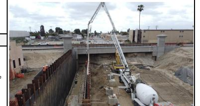
**Placement of Concrete for Retaining Walls**
